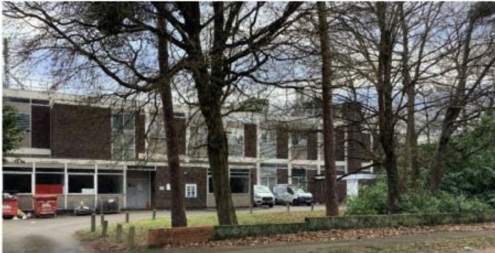
Figure 19: The Telephone Exchange (Source: South Farnborough CAAMP)
